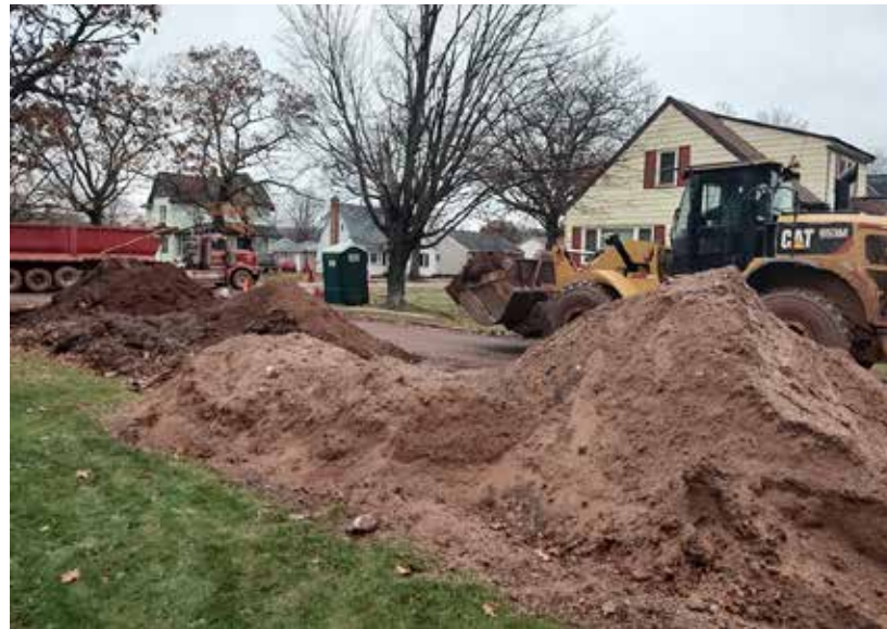
Construction in Negaunee
