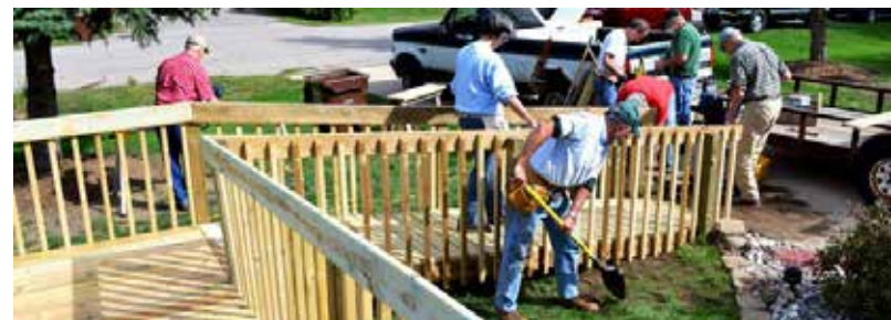
Building an Accessibility Ramp
