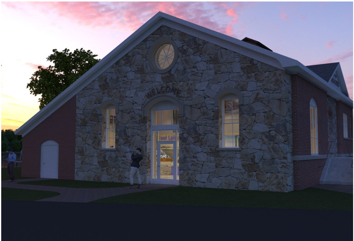
View from U.S. 41 Highway
