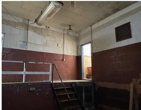
SE Corner of Mezzanine
