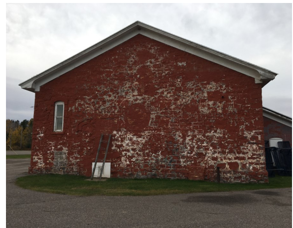
Northeast Facing Facade
