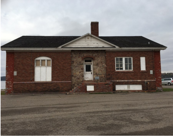
Croix Street Facing Facade
