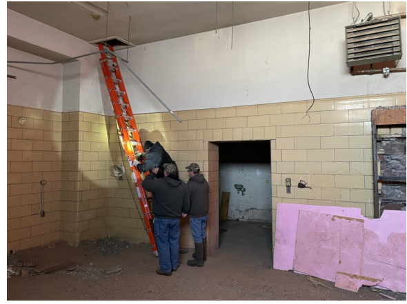
Attic Access Trap Door
