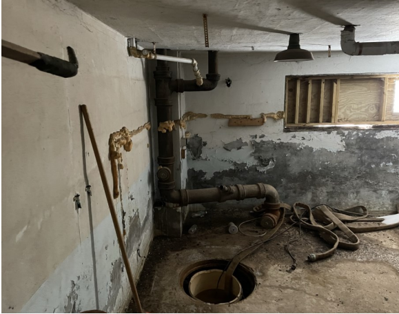
Basement Looking at Sump
