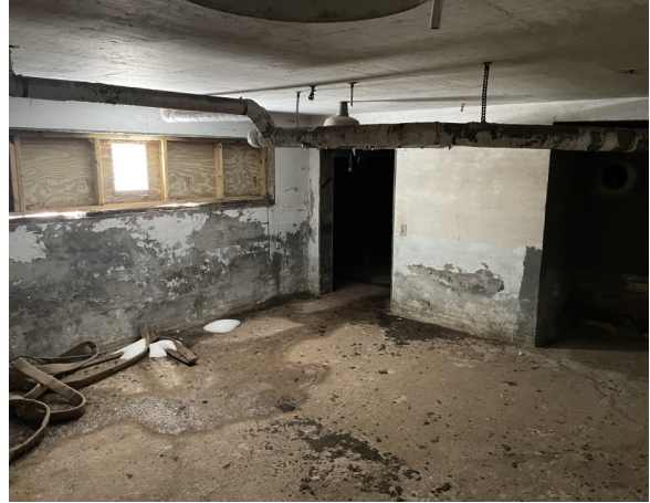
Basement Looking at SE Corner
