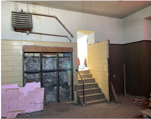
Stair down from Croix Street Entry
