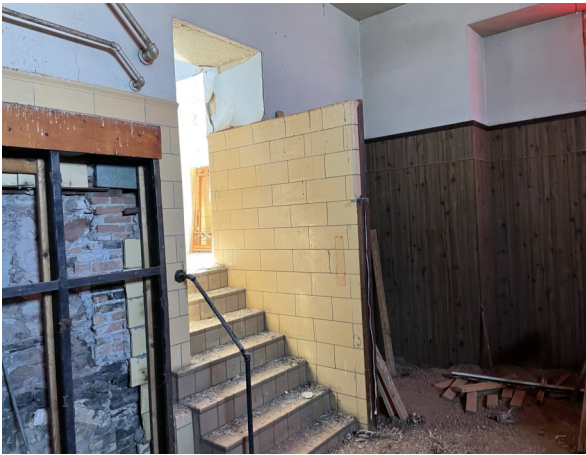
West Room - Looking at Stair to Entry
