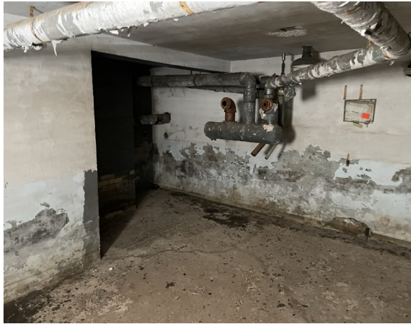
Basement Looking at SW Corner
