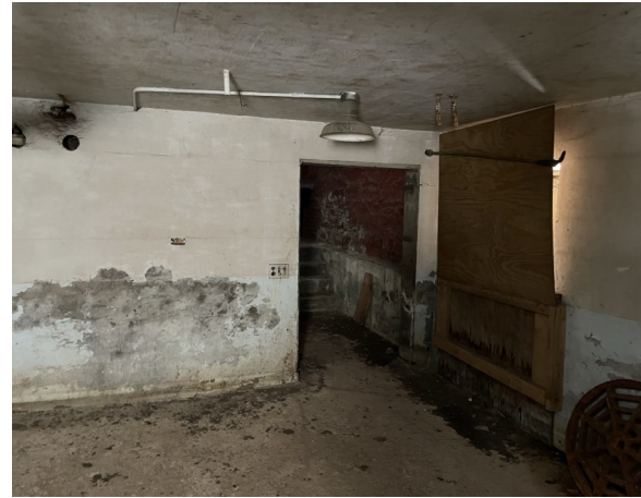
Basement SW Corner
