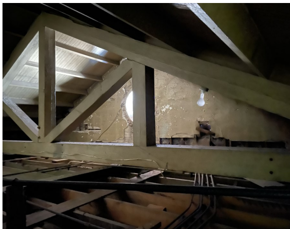
Wood Timber Truss in Attic
