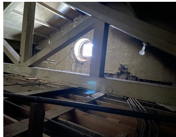
Window at Attic Gable
