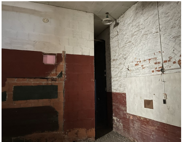
Clay Tile Wall to be Removed
