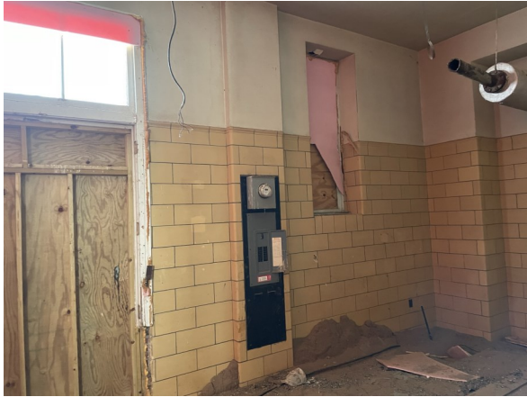
Wall Facing U.S. Highway 41
