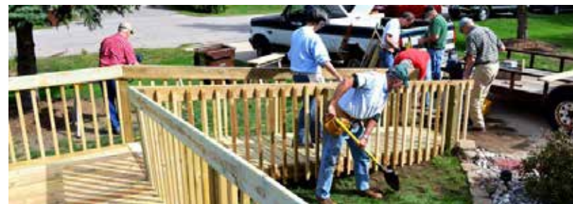
Building an Accessibility Ramp
