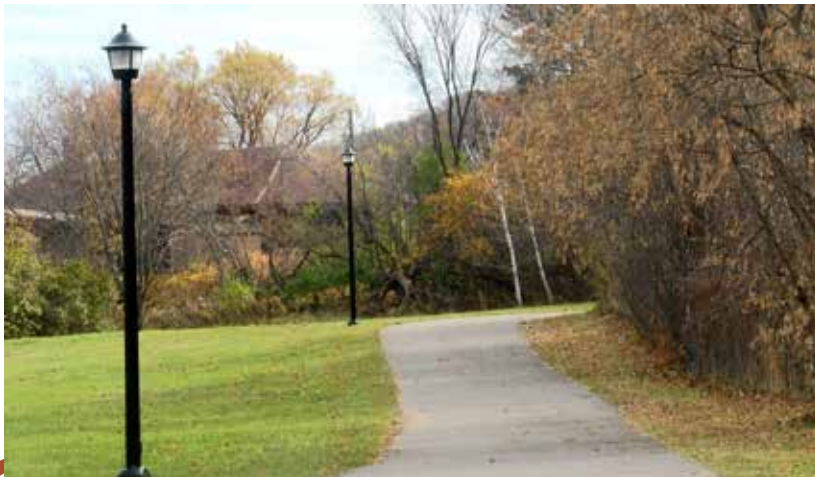
Lighting on the IOHT
