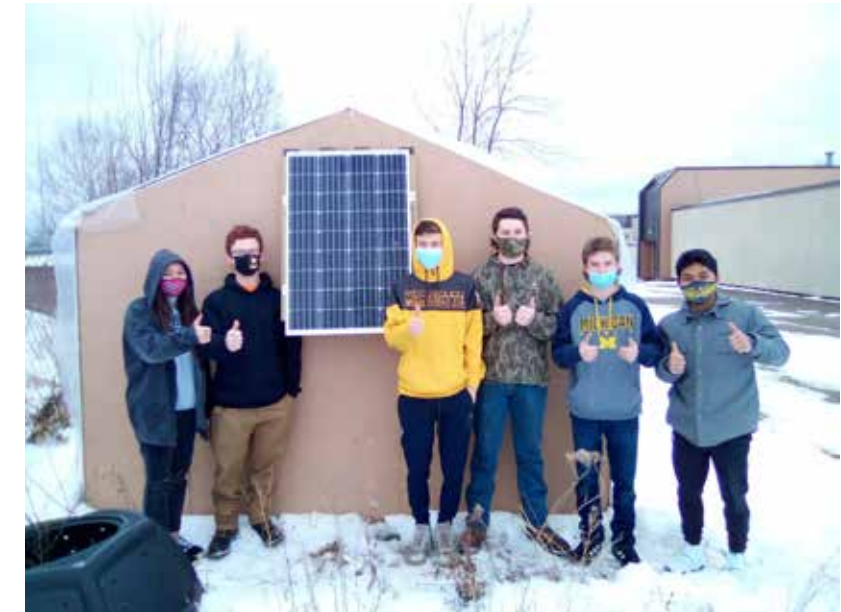
Negaunee High School Students Install Solar Panels for Project
